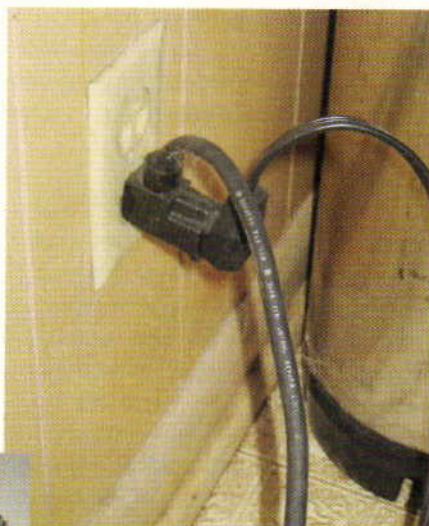
TOP: The thermostat is plugged in the wall and the freezer plugs into the thermostat.
