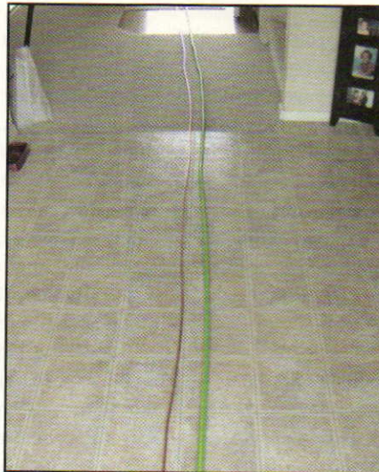
Straightening the copper tubing and hose will make inserting the one in the other easier. Use dish soap for lubrication.
